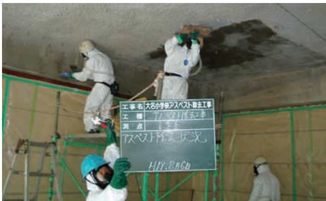
Public Work: Ona Elementary School Asbestos Removal Work
